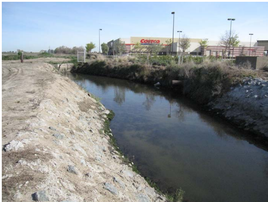
View to the north at Data Point 1. Shows the west bank in the forefront on the left side of the photo and the east bank on the right side of the photo. Note the rip-rap with a concrete pour on the east bank.
