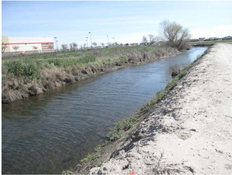
View to the south at Data Point 5. Shows the west bank in the forefront on the right side of the photo and the east bank on the left side of the photo.
