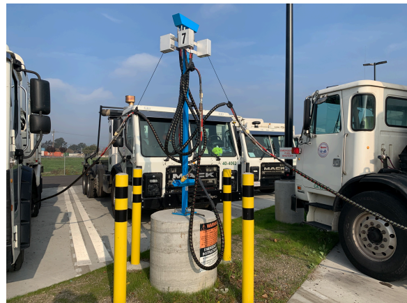
The Public (Left) and Solid Waste Division (Above) Compressed Natural Gas Dispensing Stations, Located at the Water Quality Control Facility
