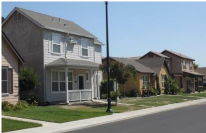
Streetscape with varied elevations
