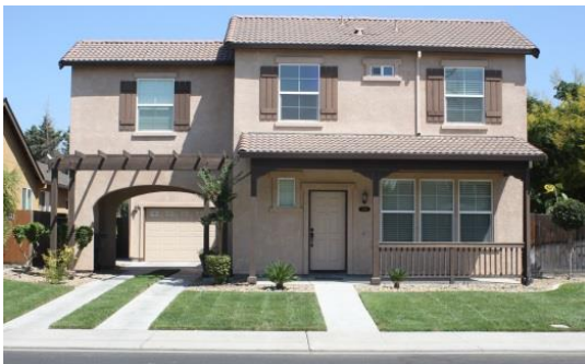
Recessed garage, shutters and porch
