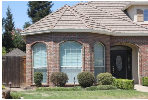
Enhance architectural window feature
