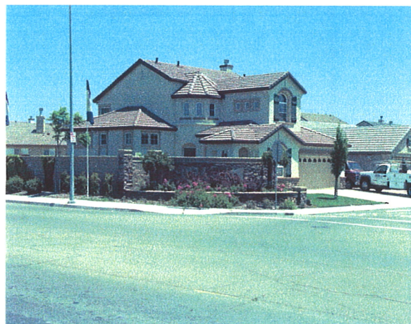
Photo 4.1-3 Residence, Villa Ticino East
