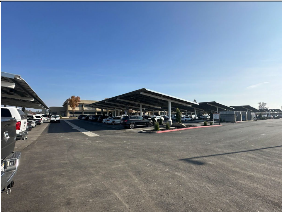
16. Facing east, the photo shows the developed parking lot along with solar structures and buildings in the background.
