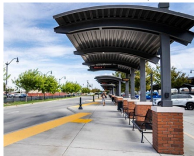
Manteca Transit Bus Bays
